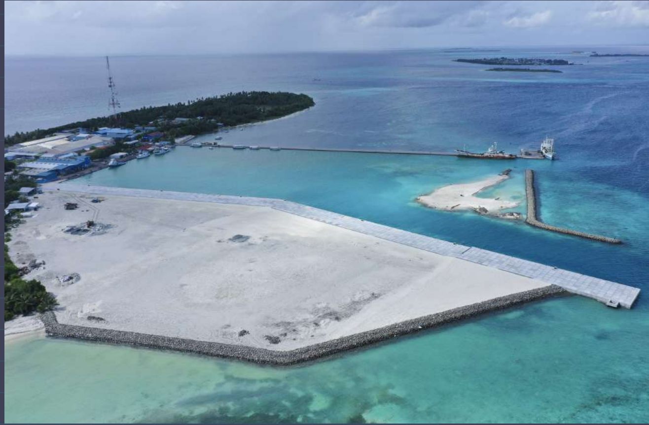
LH. FELIVARU RECLAMATION AND HARBOUR DEVELOPMENT COMPLETED DATE: 13-MAY-23
