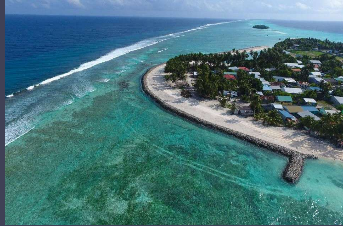
TH. GAADHIFUSHI SHORE PROTECTION STRUCTURES COMPLETED DATE: 25-APR-23
