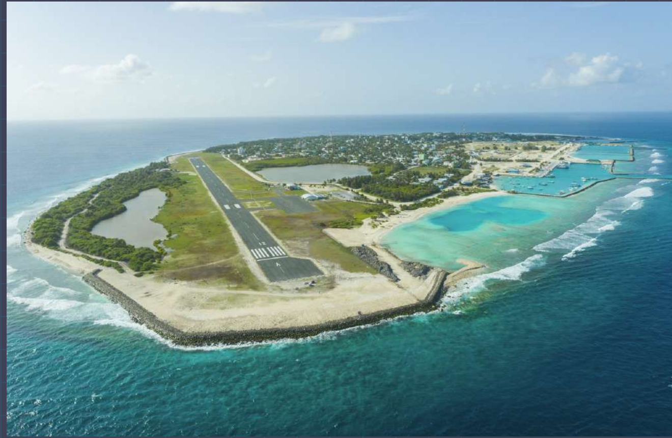
HDH. KULHUDHUFFUSHI AIRPORT SHORE PROTECTION STRUCTURES COMPLETED DATE: 14-JUNE-23
