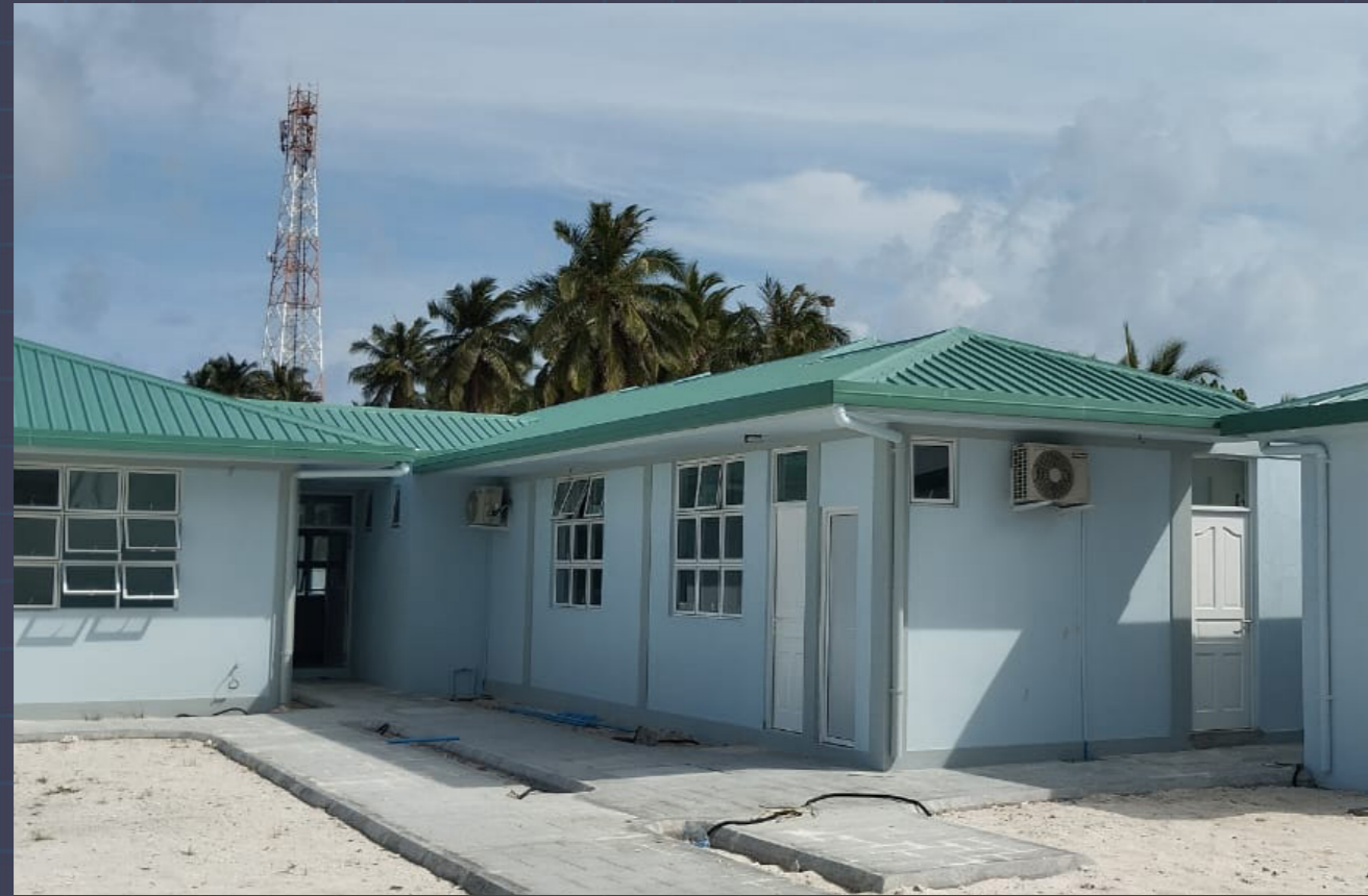
HA. HOARAFUSHI JUVENILE JUSTICE UNIT (HALFWAY HOUSE) COMPLETED DATE: 05-NOVEMBER-23
