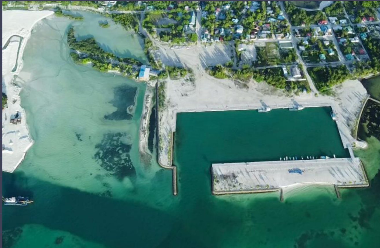
DESIGN AND BUILD OF HARBOUR CONSTRUCTION IN S. HULHUDHOO COMPLETED DATE: 15-OCTOBER-23
