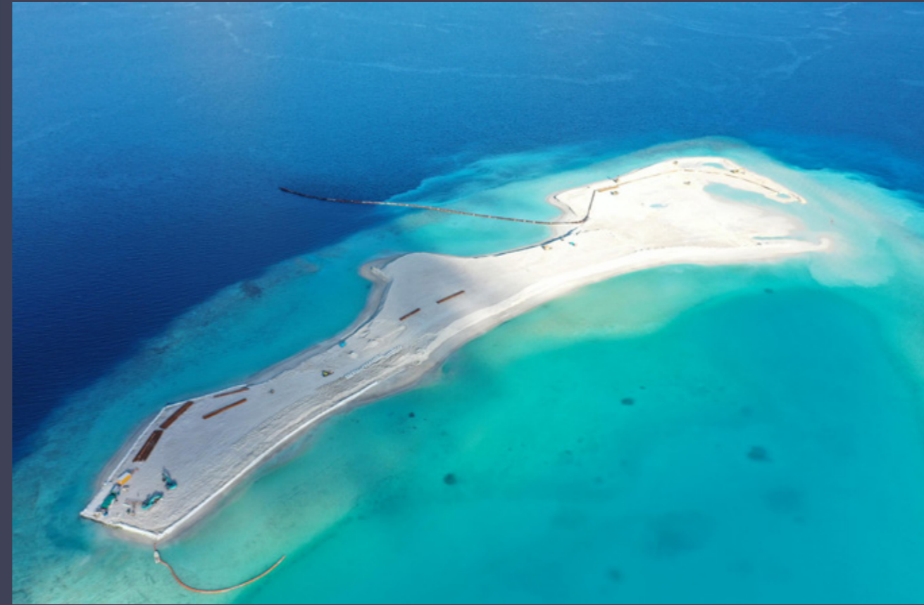
DREDGING WORKS AT NAMMOS NEDAFUSHI LAGOON COMPLETED DATE: 29-NOVEMBER-23
