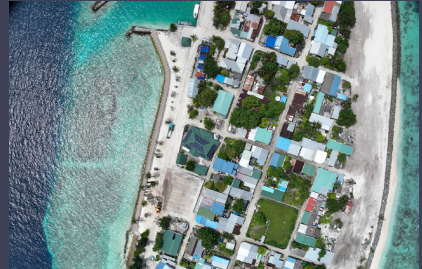
DESIGN AND BUILD OF SHORE PROTECTION STRUCTURES AT ADH. KUNBURUDHOO COMPLETED DATE: 31-OCTOBER-23
