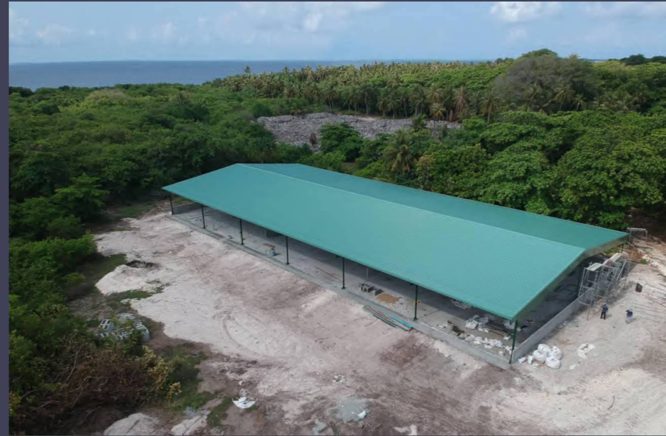
HA. IHAVANDHOO SCHOOL MULTI-PURPOSE HALL COMPLETION WORKS COMPLETED DATE: 24-JULY-23
