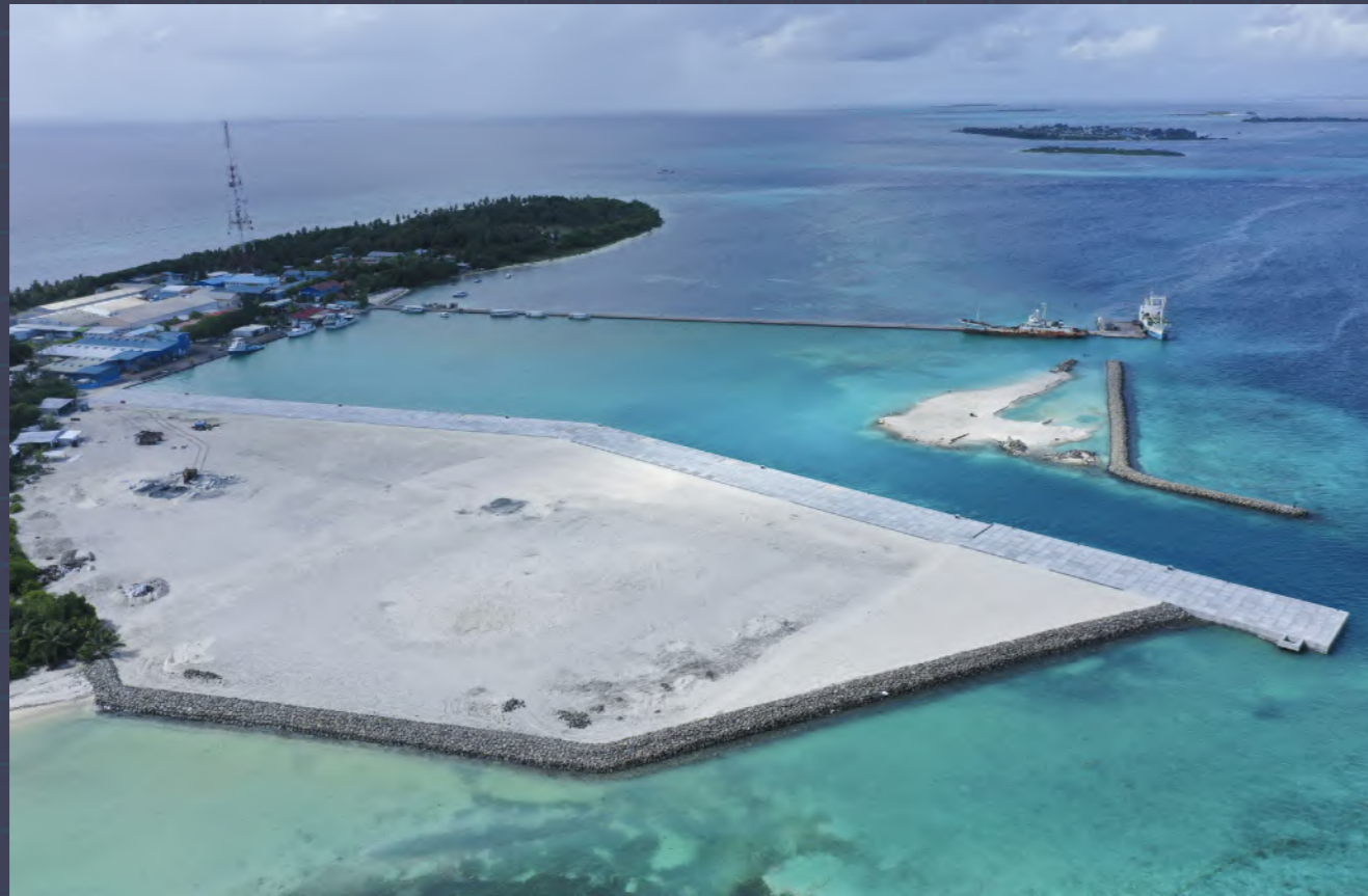
M. DHIGGARU LAND RECLAMATION AND SHORE PROTECTION COMPLETED DATE: 14-SEPTEMBER-23
