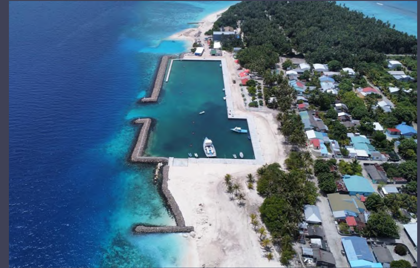
LH. HINNAVARU HARBOUR EXTENTION CONSTRUCTION COMPLETED DATE: 05-AUGUST-23
