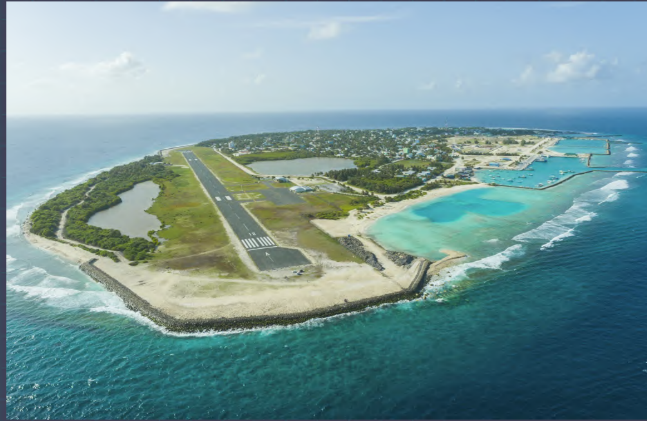
HA. HOARAFUSHI DESIGN AND CONSTRUCTION OF JETTY COMPLETED DATE: 04-SEPTEMBER-23
